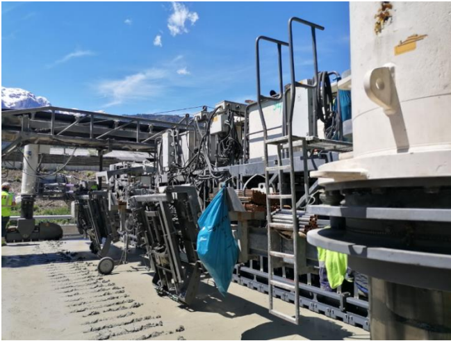
Figure 23. Automatic installation of anchors and dowels, Source: K. Hrapović, 2021
