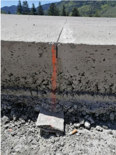
Figure 20. Flat drain under concrete pavement, Source: K. Hrapović, 2021
