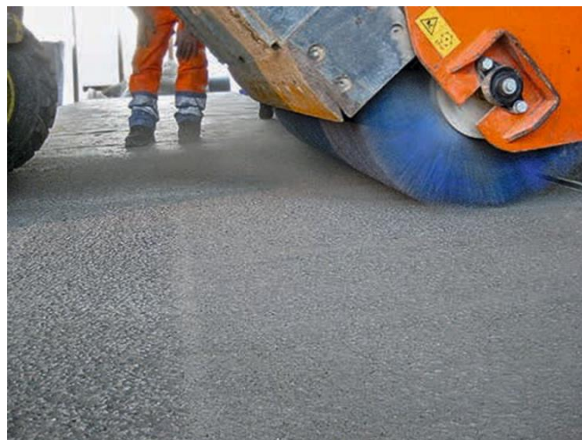
Figure 30. Brushing out the surface, Source: G. Müller, 2015
