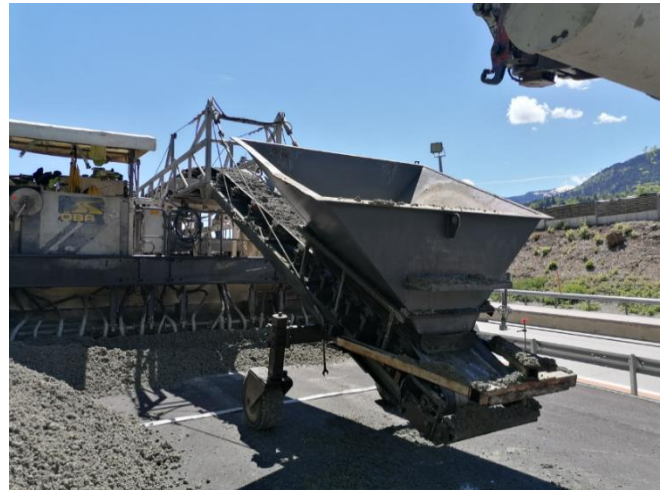
Figure 15. Transfer hopper for top concrete, Source: K. Hrapović, 2021
