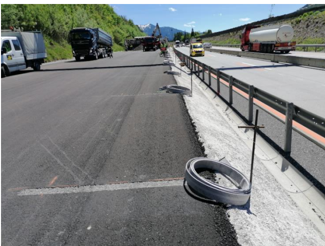
Figure 17. For flat drainage, lightly milled bituminous base of asphalt AC16 trag 70/100, T3, G4 under concrete pavement, Source: K. Hrapović, 2021
