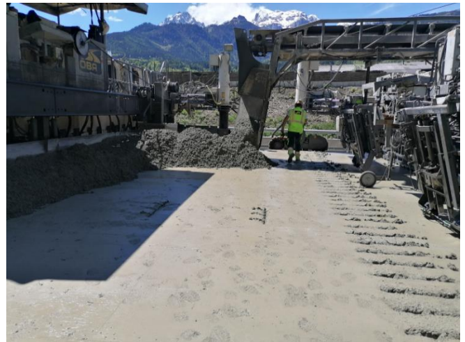
Figure 24. Installation of top concrete, Source: K. Hrapović, 2021
