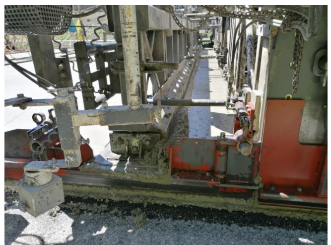
Figure 26. Vibrator for top concrete, Source: K. Hrapović, 2021
