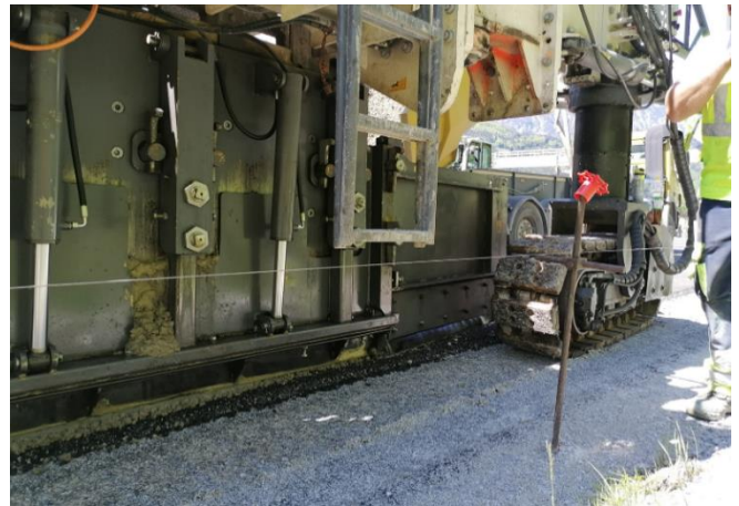
Figure 21. Paving of the bottom concrete, Source: K. Hrapović, 2021
