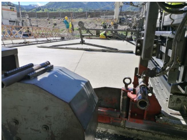
Figure 27. Lengthwise smoother for top concrete, Source: K. Hrapović, 2021
