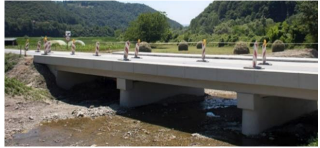
Figure 4. Rehabilitation of bridge after floods, EU donation [9]
