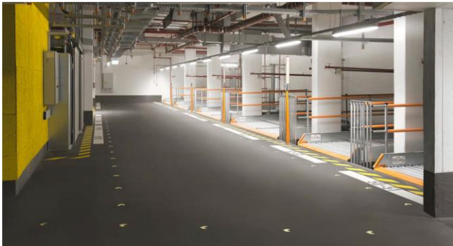
Figure 19. Stacking car park with pit in a multi-storey car park Source: BGA 2021
