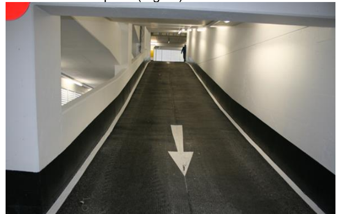
Figure 17. Interior ramps with protective or levelling layer on waterproofing + 3.00 cm ribbed mastic asphalt Source: Felsing & Piring 2016a
