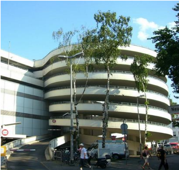
Figure 7. An example of spiral ramp: Spiral driveway to a multi-storey car park in Braunschweig, Germany Source: Wikipedia 2022
