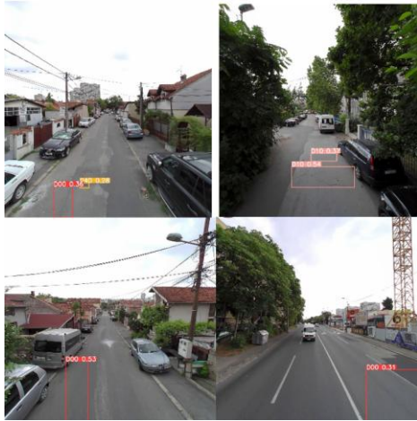
Figure 11. Examples of road distress: longitudinal cracks and potholes (upper left and lower right), transversal cracks (upper right) and alligator cracks (lower left)
