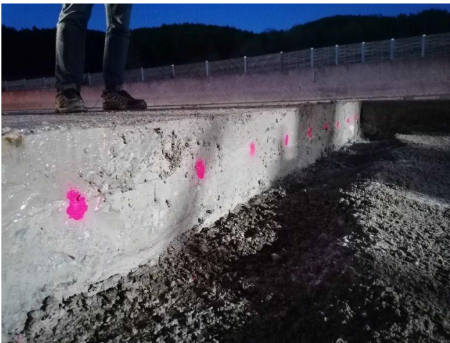
Figure 14. Marking for drilling for the adhesive anchors Source: Author 2021
