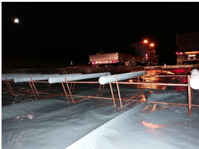
Figure 19. Dowels laid on baskets in the area of the dummy joints Source: Author 2021
