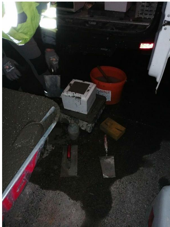
Figure 22. Concrete testing: Production of a cube- shaped test specimen for subsequent laboratory testing of the cube compressive strength f_{c, cube} of the concrete Source: Author 2021
