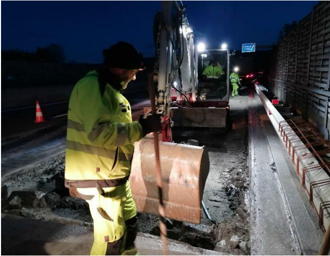
Figure 13. Removal of the remains by means of an excavator bucket Source: Author 2021
