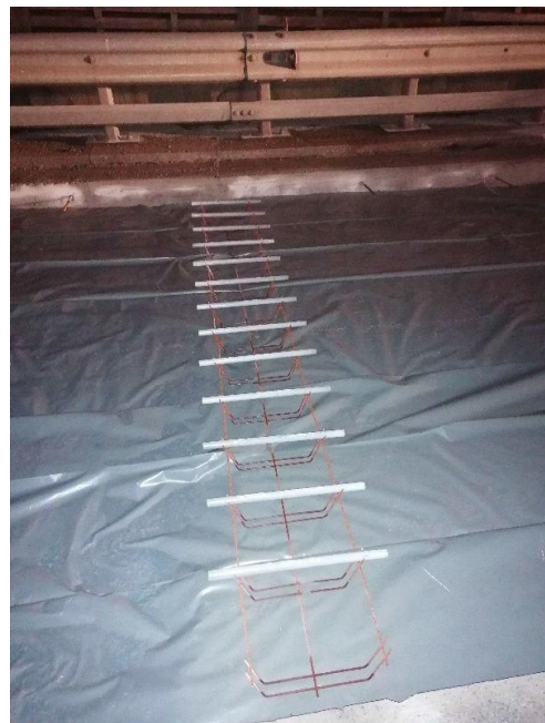
Figure 18. Dowels laid on baskets in the area of the dummy joints Source: Author 2021
