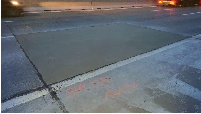
Figure 24. Finished concrete slab after traffic clearance the next morning after a long night Source: Author 2021
