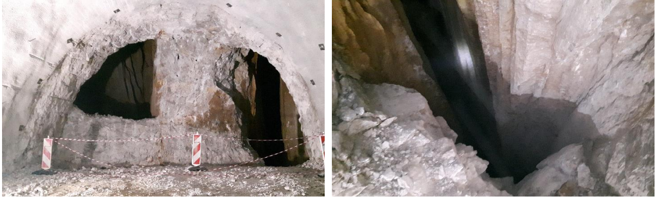
Figure 1a & 1b. 1a. Tunnel face at km 22+220 on the left side, 2b. Look into the cave on the right side Source: Face mapping reports
