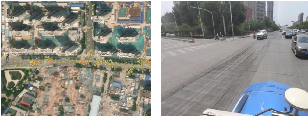
Figure 3. Road section No.14900778
