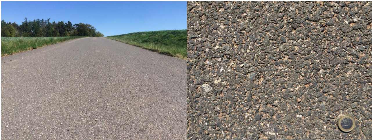
Figure 4: The mixture containing 50% RA with rejuvenator during laying
