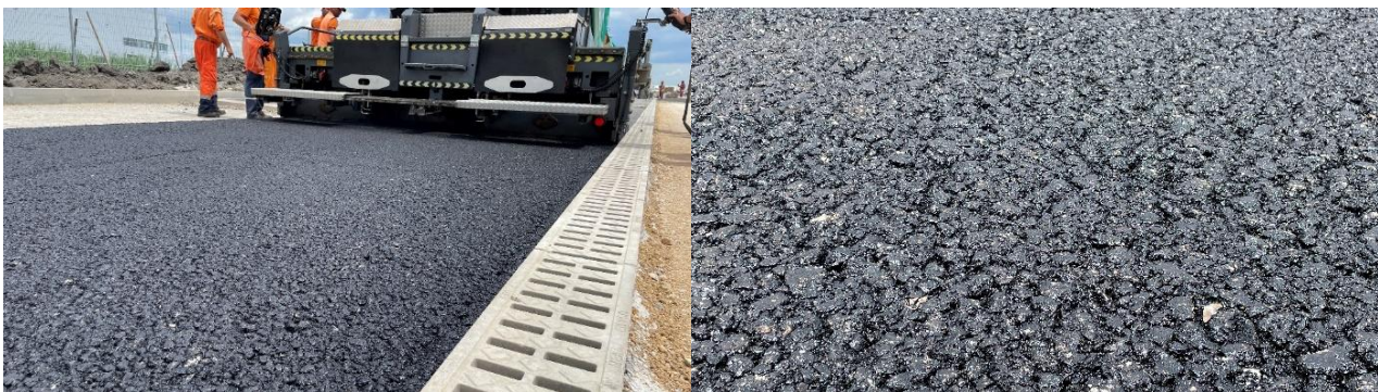
Figure 3: The mixture containing 40% RA with rejuvenator during laying
