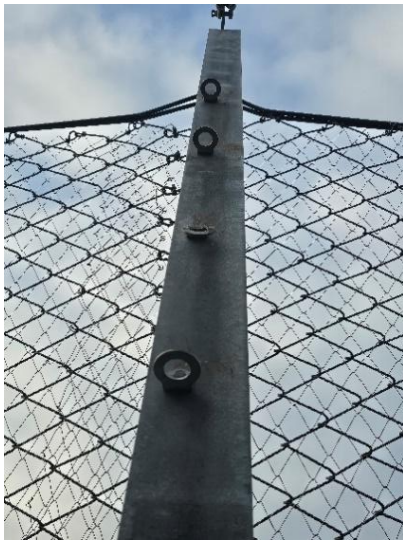
Figure 15. Detail of the approved anchor points on the back of the GBE-2000A post (Table 4.)
