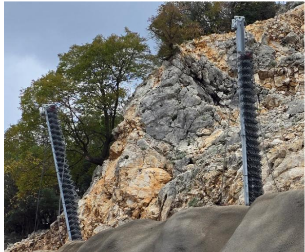
Figure 16. Detail of modular posts with pre-assembled mesh for easier installation
