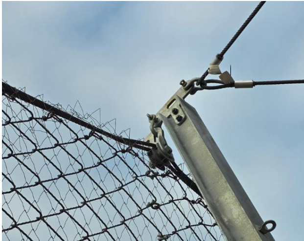
Figure 13. Detail of the head of a GBE-2000A intermediate post (piece 1)
