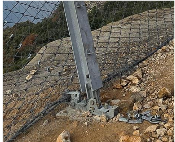
Figure 14. Detail of the foot and base plate of a GBE-2000A
