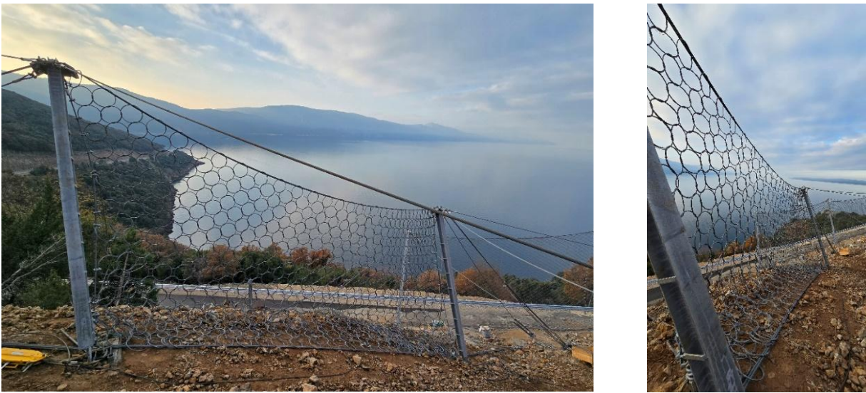
Figure 18. Finished product, ROCCO 2000 one-field barrier system
